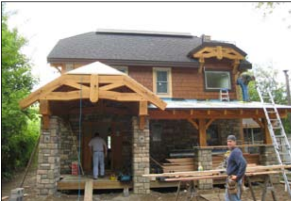
Front Elevation - Under Construction
