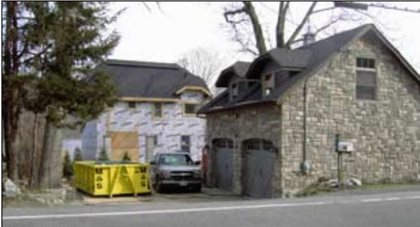
Front Elevation - Under Construction
