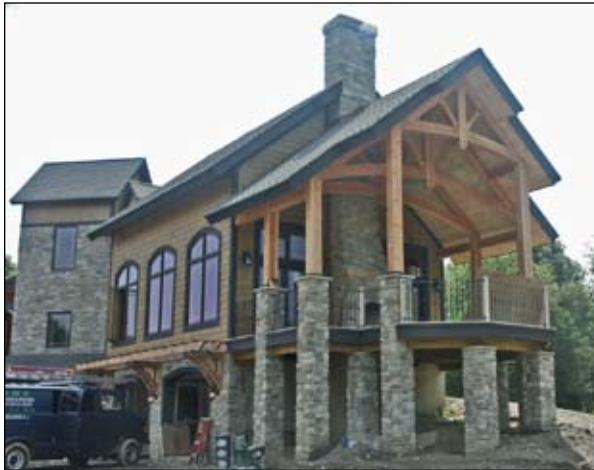
Exposed Timber Frame Veranda & Stone Fireplace
