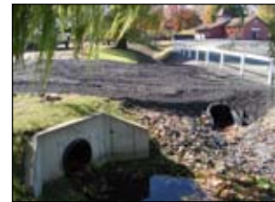
New Drainage Piping & Bridge
