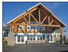
Front Entrance - After
