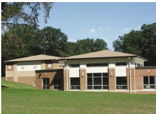
Gymnasium/ Media Center elevation.
