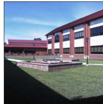
Classroom Wing Addition
