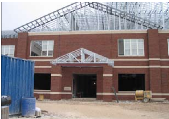
Memorial School - Under Construction
