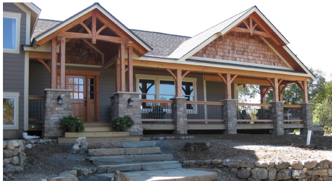
View of the new front entry porch.
