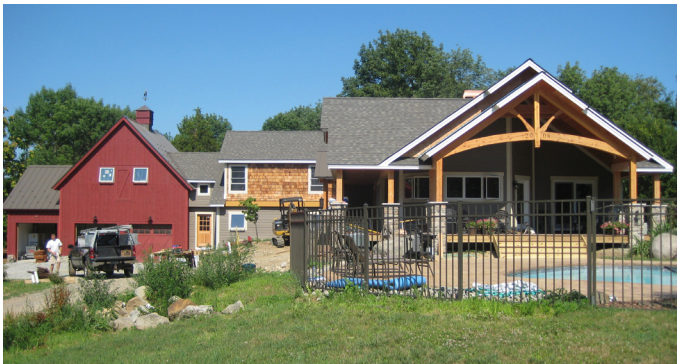
View of the front elevation.
