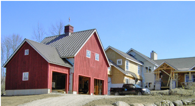
View of the front elevation under construction.
