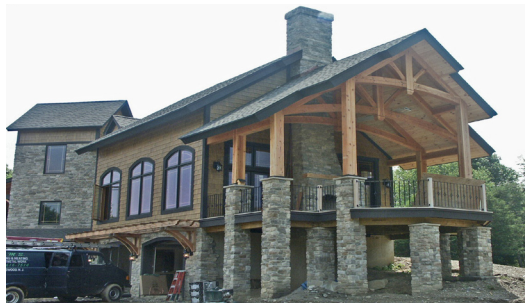
View of the Great Room and Veranda addition.
