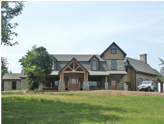
View of the renovated front elevation.
