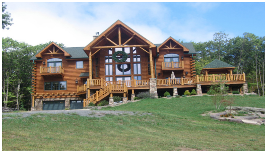
View of the exterior of the house.
