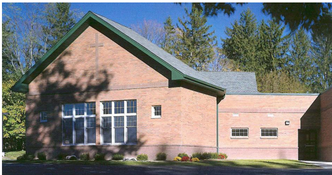
Overall view of the completed classroom and library addition.
